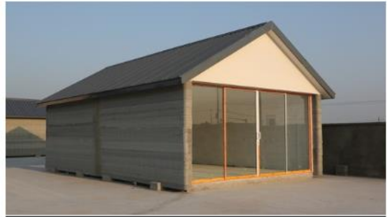
Small home constructed from 3D-printed building blocks (Image: Winsun New Materials) Image Gallery (3 images)
